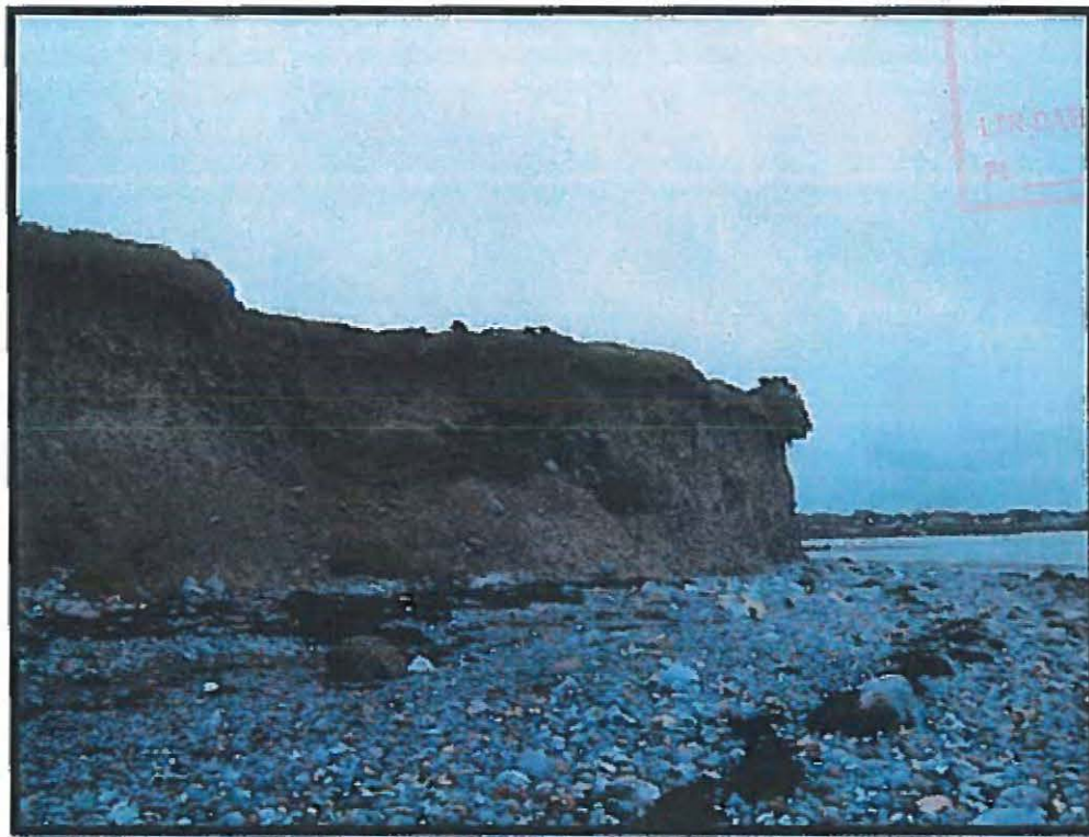
View of eroding cliff face from foreshore
